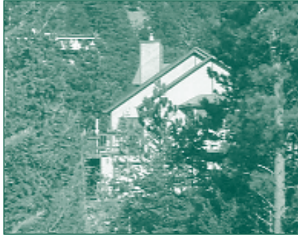
Combustible House with no Defensible Space
