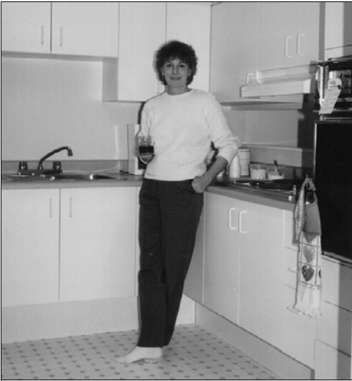
Adjustable lower cabinets, removable doors & shelves below sink & cooktop, installed for a standing cook.
