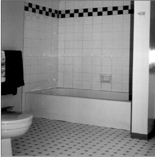
New tub ready for grab bar placement or conversion to shower. Tiles cover floor under tub, whole floor slopes to tub drain.
